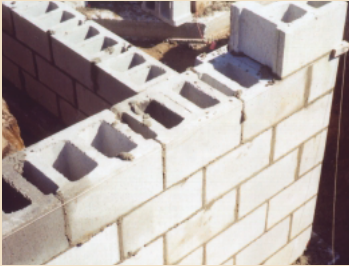
Multiple courses allow easy construction of 9' basement walls.
