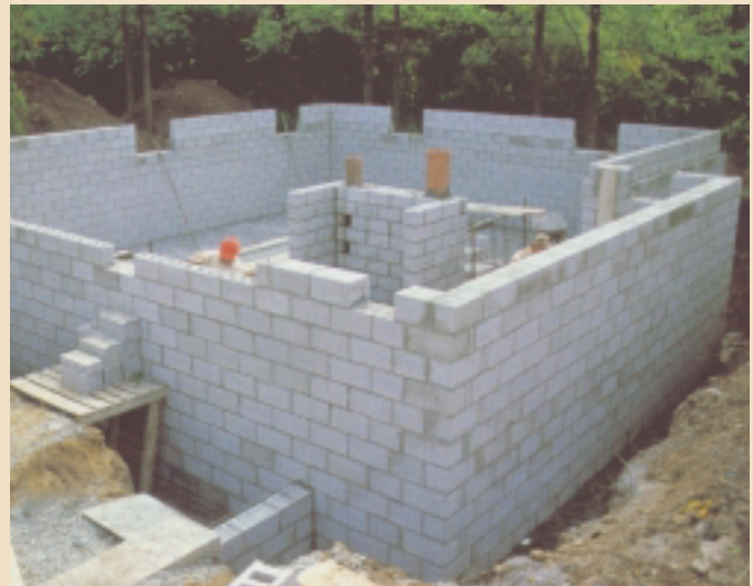
Once foundation walls are constructed and mortar cured, backfilling may commence.
