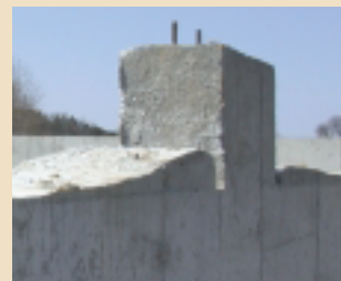
Poured foundation wall requiring further finishing.
