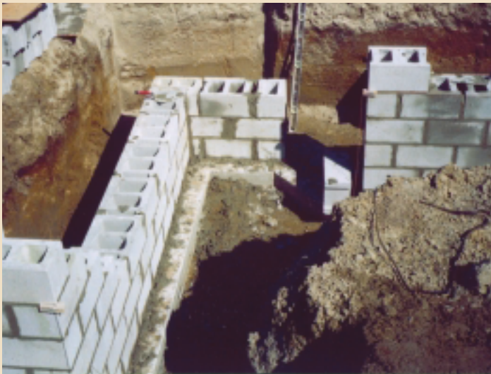
Concrete masonry allows easy design flexibility without the need for custom forms.
