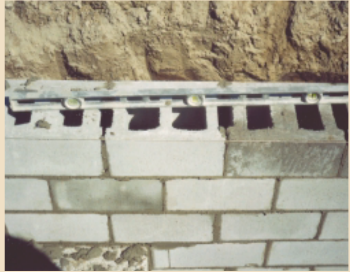
Level and true foundation walls provide ideal sills for floor joists and framing.
