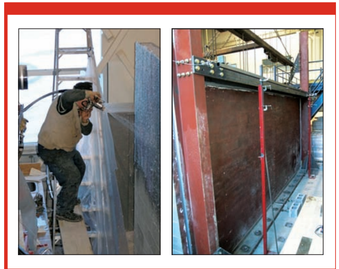
GFRP-sprayed hollow concrete block wall testing at the University of Calgary. This reinforcing method could be a good option.
