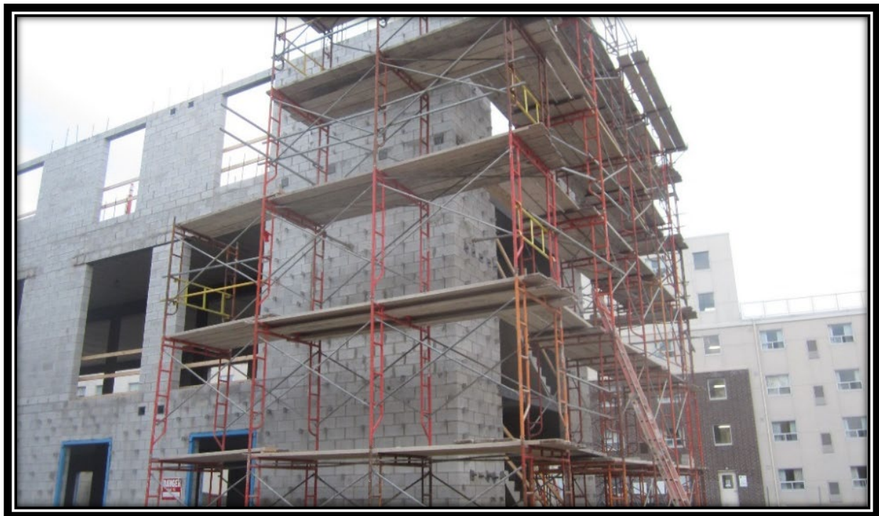
Figure 2 - Loadbearing masonry walls can be used for interior and exterior walls.
