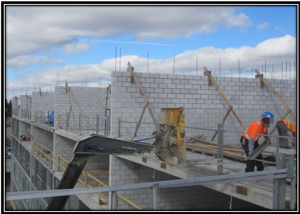
Figure 1 – Unit demising walls built out of loadbearing masonry provide excellent fire rating and sound proofing as well as being the main structural element of the building.
