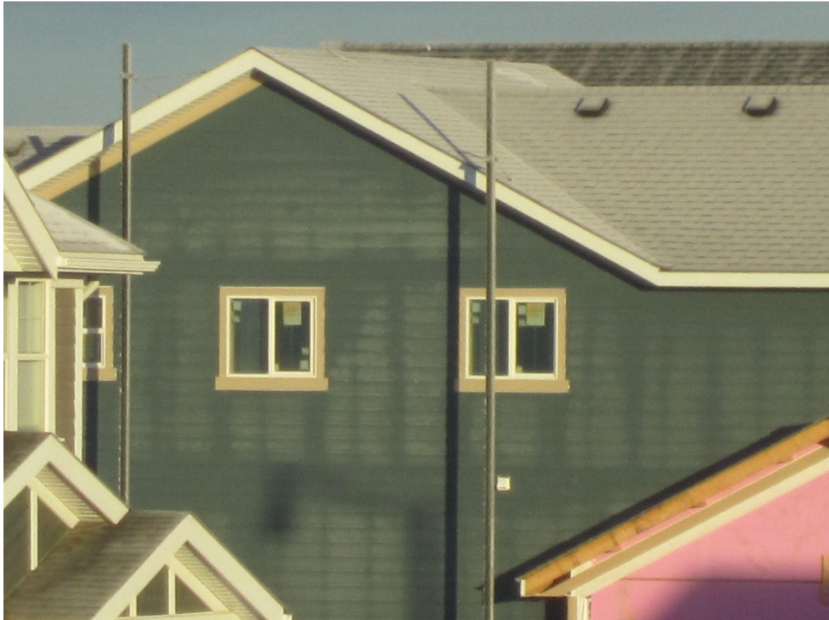
FIGURE 4: Thermal bridging of a wood-stud wall evidenced by dark areas on white frost at locations of the wood framing. 40
